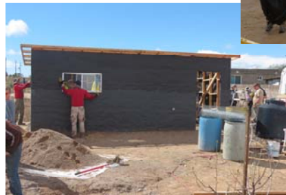
Day 3, 2nd coat of stucco and roofing
