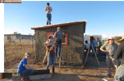
Day 3, 2nd coat of stucco and roofing
